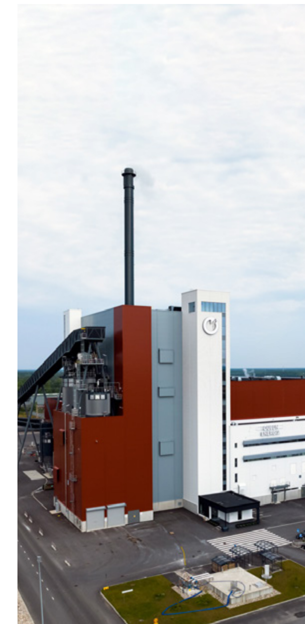
Laanila Biopower Plant
